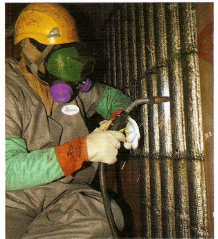
Fig. 2 — Inconel cladding protects the tubes that make up the boiler, extending their lives from 3 to 15 years. To maintain the proper dilution rate, GMAW-P is used.
