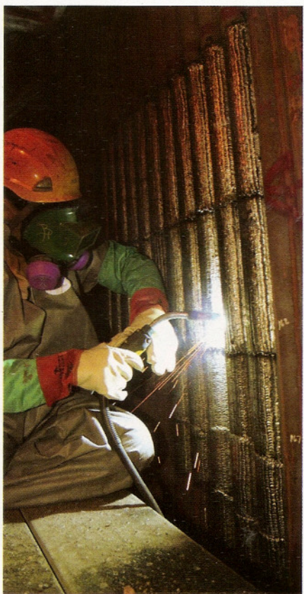
Fig. 5 — Welders become productive more quickly with the newer pulsed equipment because setup is quicker, less complicated, and requires less training, noted Brad Hooper, supervisor, Northeast Regional Maintenance, Covanta Energy.
