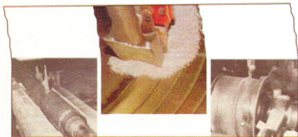
Fig. 2 — Submerged arc welding of rolls.
