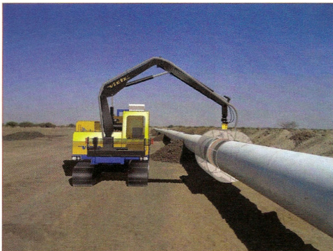
Fig. 3 — The VIETZ pipeline laser (VPL) system. (Photo courtesy of VIETZ GmbH.)
